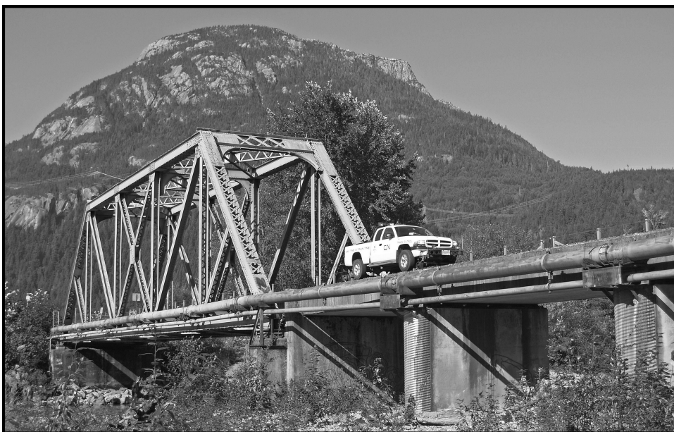
Another truss span from the 1907 Pitt River railway bridge found a new home on the PGE after its days as part of the 1915 road bridge were over. After five years in storage at Squamish, it was installed over the nearby Mamquam River in 1962. Following flood damage in 1976, the truss span was flanked by eight pre-stressed concrete box girders, as seen here on September 2, 2006, with a CN hi-rail pickup truck making a northbound track patrol ahead of a train. (Photo by Ian Smith)
