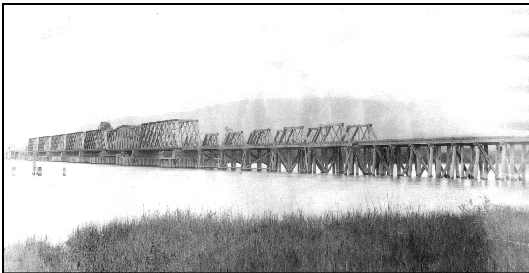
The first rail crossing of the Pitt River was this wooden pile and sawn timber structure completed in late 1883. The view is from the east bank, slightly downstream of the bridge, looking northwest. The swing-span is flanked by five through-truss spans on the west side and a through-truss span and five pony-truss spans on the east end. (City of Vancouver Archives CVA 3-37)
