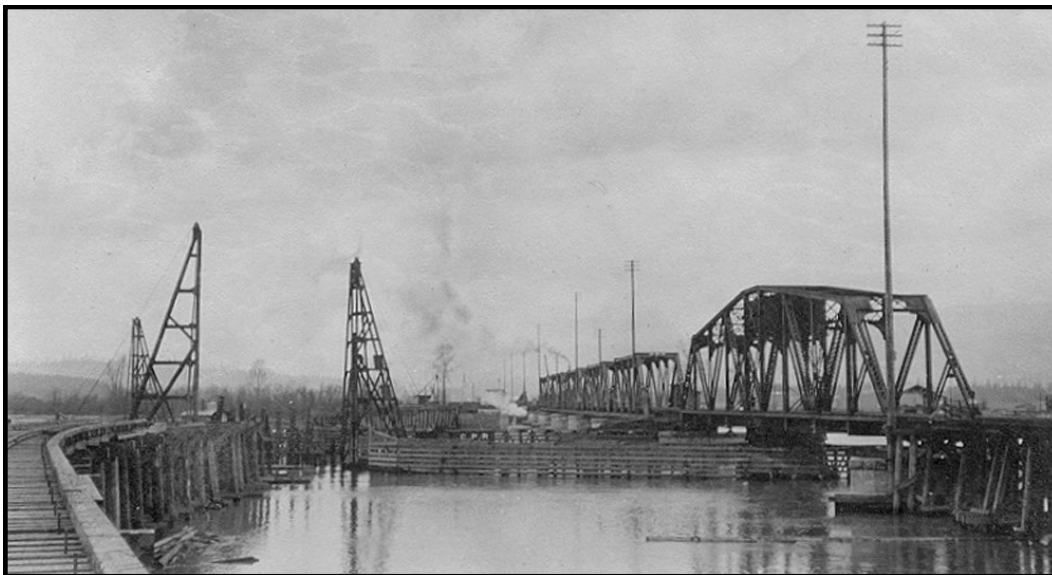
This photo taken in the spring of 1913 illustrates the location of the third bridge in relationship to the 1907 bridge. The view is looking west from a partly-built falsework trestle that will support the steelwork of the double-track bridge as it is being assembled. The 1907 bridge is at right. (Author's collection)
