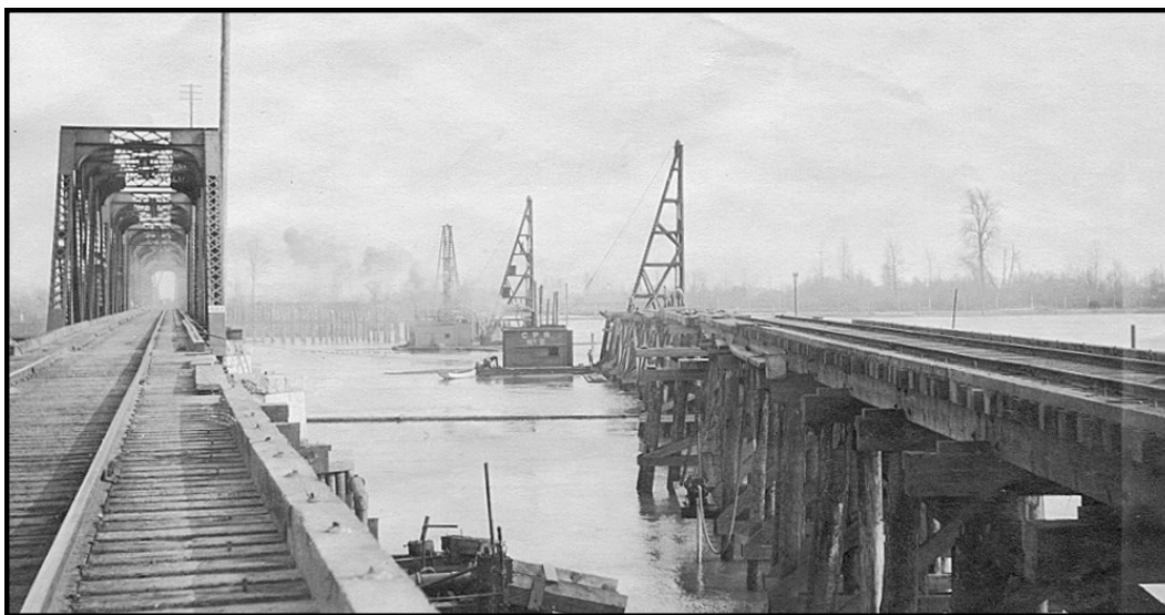
In this view, taken at the same time in the spring of 1913 as the photo on page 9, the photographer is standing on the 1907 bridge, looking east across the river, with the falsework trestle for the new bridge at right. Work on a temporary bypass trestle farther to the right has yet to be started. (Author's collection)
