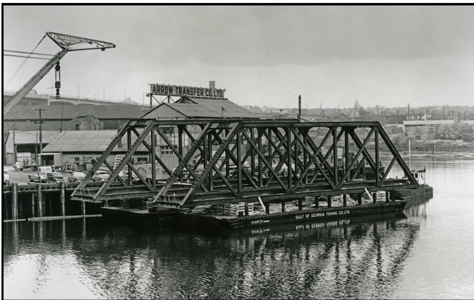
On May 31, 1957, soon after their 42-year life as part of a road bridge had ended, two truss spans of the 1907 Pitt River railway bridge sit on barges tied up at the Arrow Transfer Company dock on Vancouver's False Creek, awaiting yet another relocation, this time to the Pacific Great Eastern Railway. One of these spans went to Furry Creek near Britannia Beach and the other to the Pine River crossing in the Peace River District. (Photo by Bob Harris)
