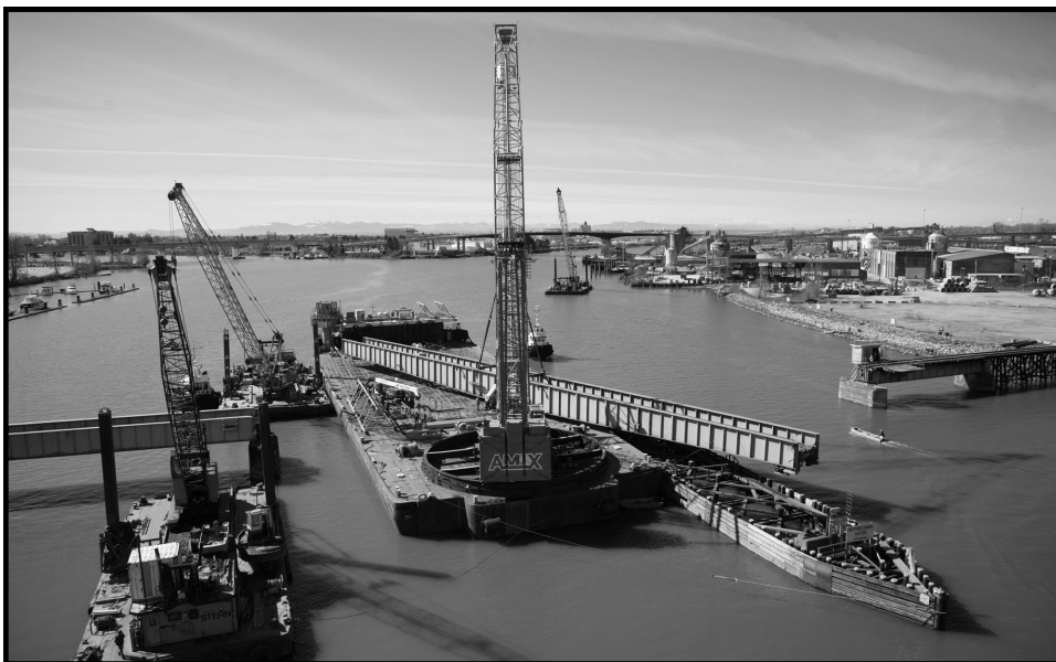
In action seen looking west from the Oak Street Bridge on March 17, a heavy crane has lifted the Marpole Bridge swingspan off its damaged pier at right, and will next transfer it on to another barge. (Photo by Corwin Doeksen)
