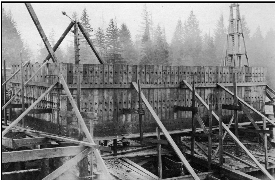
This photo of a caisson under construction shows the steel cutting edge at its base. Once the caisson has fulfilled its purpose in reaching bedrock, it will be abandoned around the base of the pier it helped to create. It will then be buried in rip-rap dumped from the finished bridge to protect the pier against river scour.
