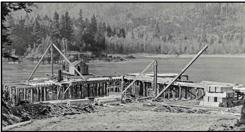
A pile driver can be seen at work building the pile trestle across the Fraser River in the early stages of construction of Hope Bridge. The view is from the Hope side of the river, with the river flowing from right to left. The photo was taken December 21, 1913, by a staff member of Armstrong, Morrison & Co., the bridge substructure contractor.
