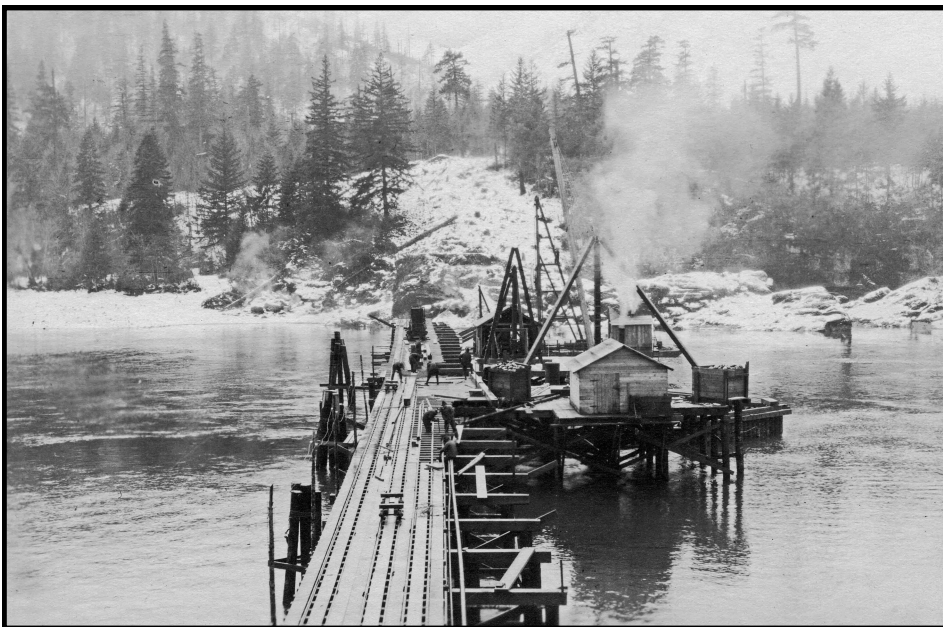
This photo looks toward the Fraser River's north bank and was probably taken from one of the pile drivers used in construction. It is dated February 1914 and was likely taken immediately after the falsework trestle was struck by floating ice on February 11, judging by the slight misalignment of the trestle at the far end, beyond the caisson for Pier 3. Note the caissons in the river to the right of the trestle.
