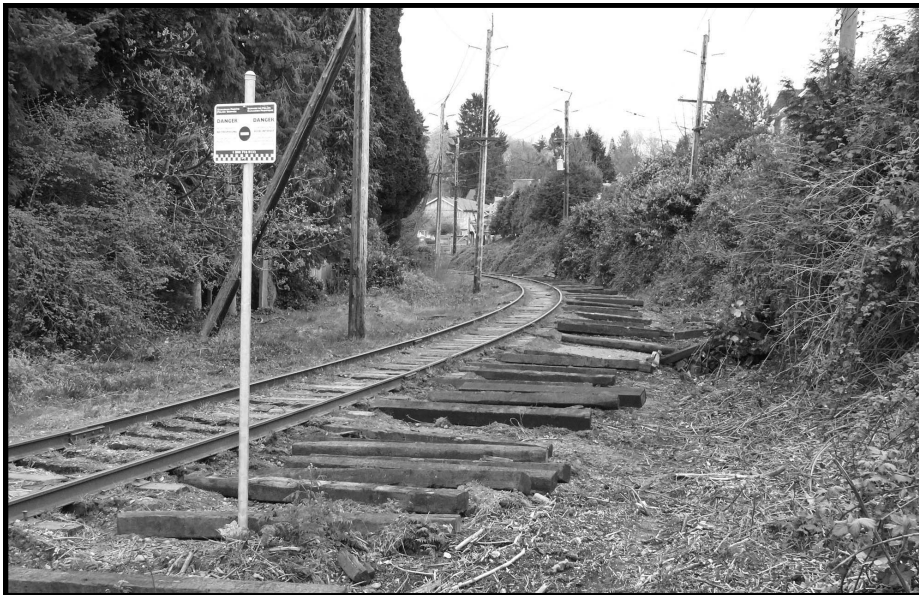
Replacement ties are laid out beside the Arbutus Line awaiting installation, in this view looking downgrade toward West 33rd Avenue on April 3 this year. Most of these have been recycled from earlier use.
