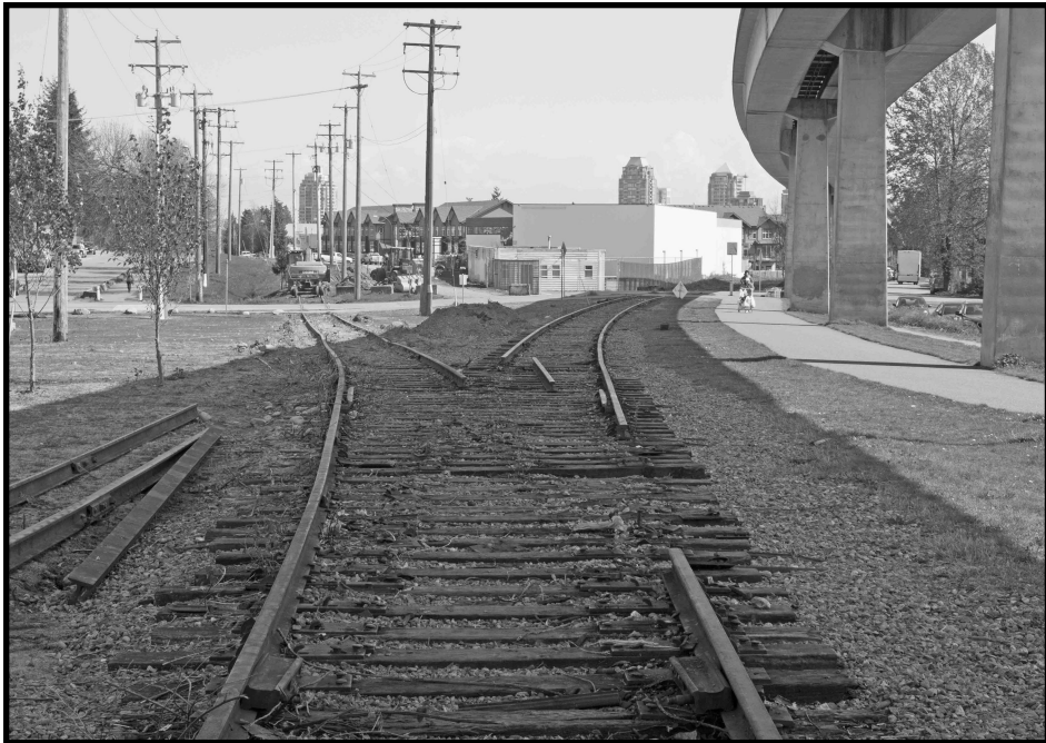
The original W&VT route to New Westminster diverges to the left, while the 1912 line curves to the right, in this scene of the track lifting work on April 8, looking east. Highland Park station lay just beyond the junction.
