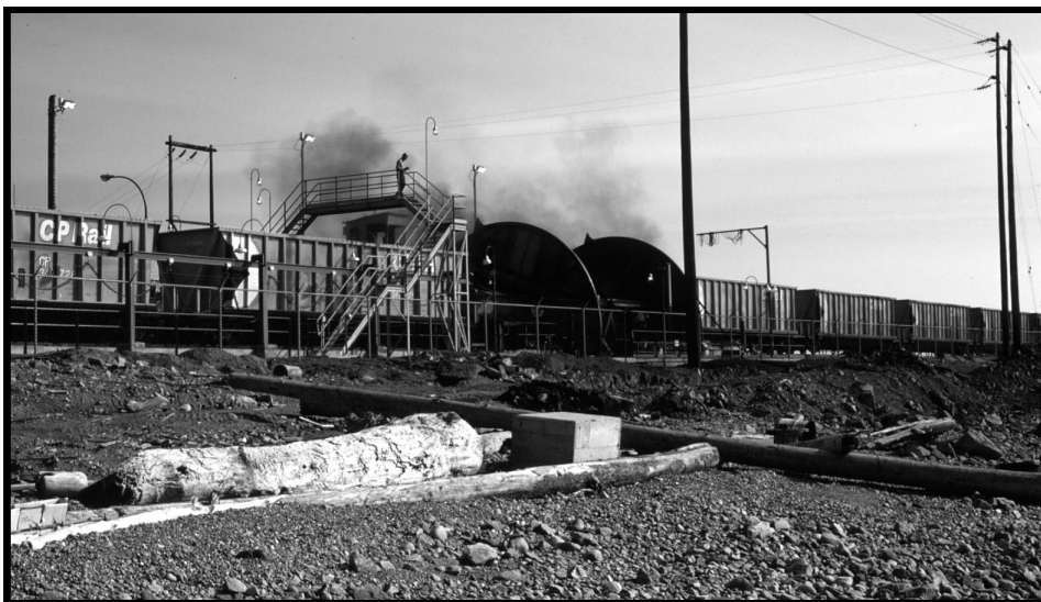
A CP unit coal train passes through the single-car, open-air rotary dumper at Roberts Bank on May 2, 1970, just days after operations began there. The two dumpers in use today are both enclosed within structures. (Photo by Dave Wilkie, WCRA Archives)
