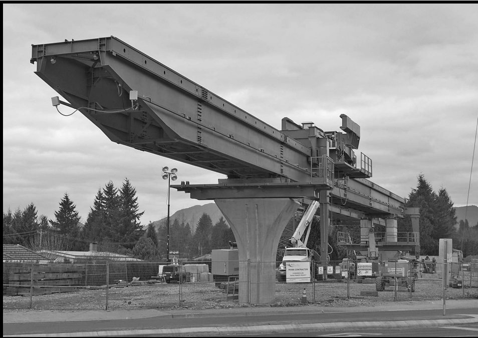
Assembly of the launching girder was well advanced in this scene on November 28 at the northwest corner of Como Lake Avenue and Clarke Road. From here it will work south on Clarke and North Road. (All photos by Ian Smith)
