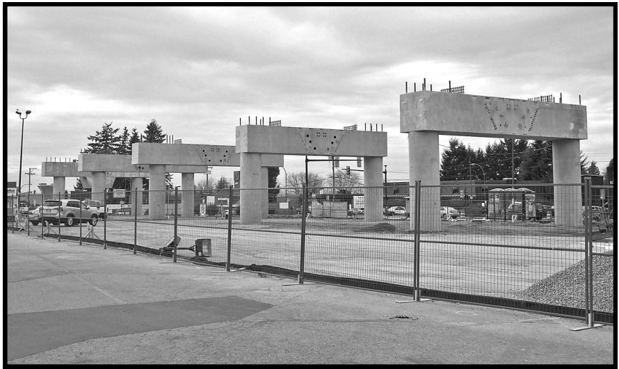
Five support beams for Burquitlam Station stand ready for the launching girder and installation of guideway segments, in this view looking southwest from the parking lot of Burquitlam Plaza on November 28. Below, grading is in progress for the at-grade guideway approaching the future Moody Centre Station, looking east on October 22. To the right is the condensed West Coast Express parking lot; three extra lots have been created to make up for the lost spaces.
