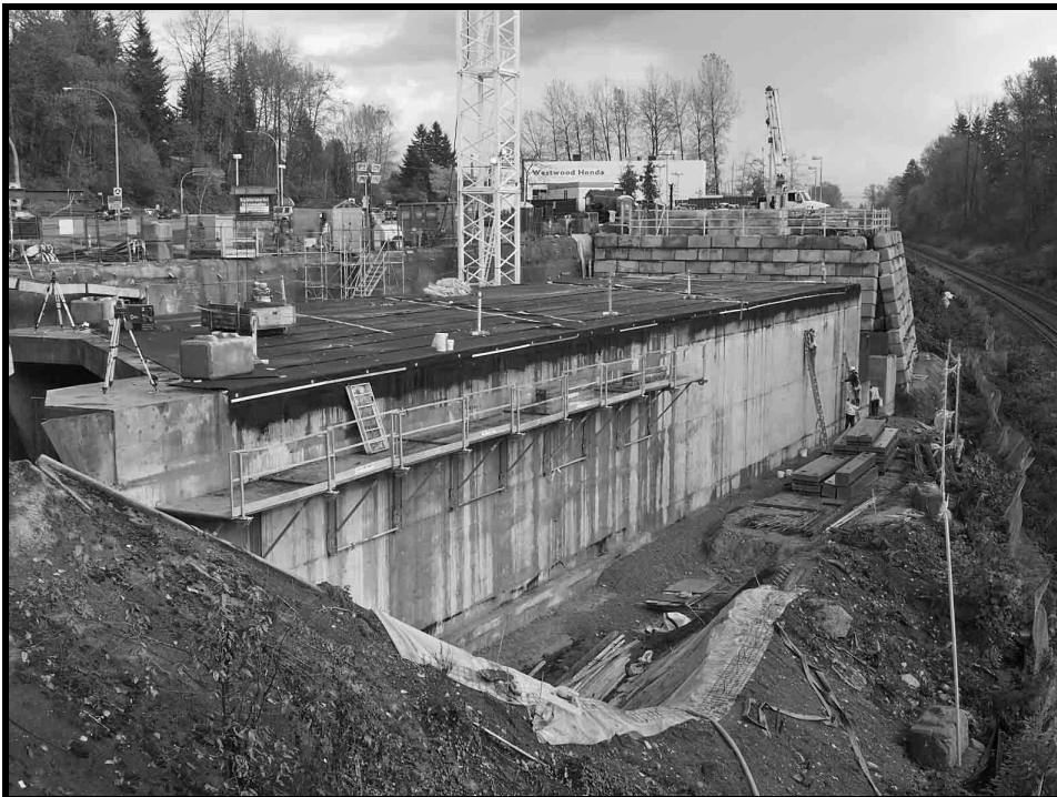
Before: This rectangular concrete box to house the platforms and running lines at Inlet Centre Station was cast in place on the east side of the Barnet Highway overpass in Port Moody, as seen on November 8. Some 50 metres long, it weighs in at 4,000 tonnes.
