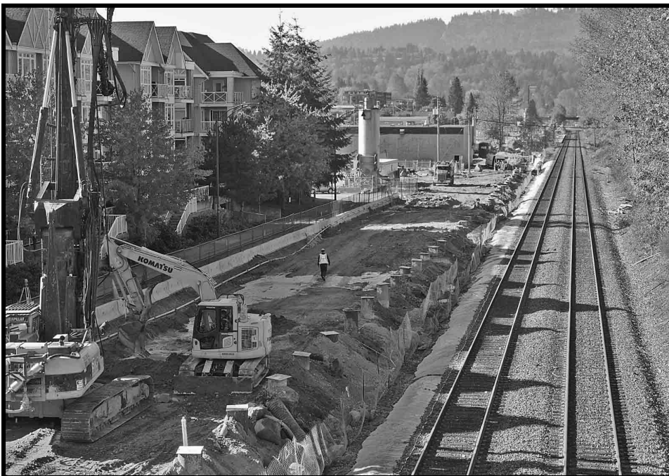
The view west from a footbridge in Port Moody on October 22 shows grading work in progress for an at-grade section of guideway, running parallel to the double-track mainline of CP's Cascade Subdivision.
