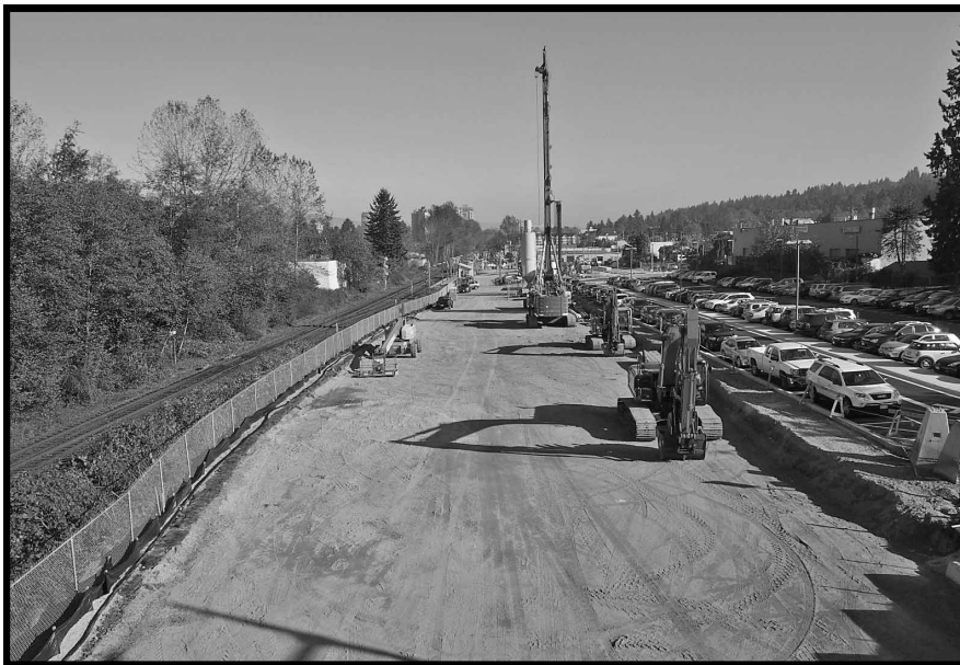
Five support beams for Burquitlam Station stand ready for the launching girder and installation of guideway segments, in this view looking southwest from the parking lot of Burquitlam Plaza on November 28. Below, grading is in progress for the at-grade guideway approaching the future Moody Centre Station, looking east on October 22. To the right is the condensed West Coast Express parking lot; three extra lots have been created to make up for the lost spaces.
