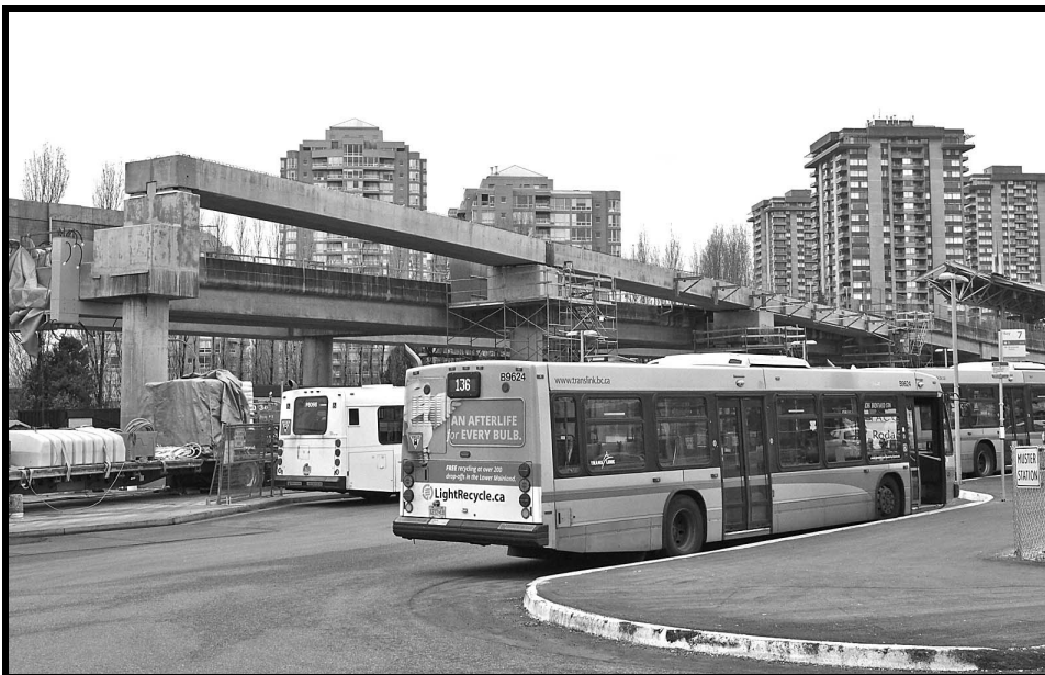
At the junction with Millennium Line, three spans have been placed atop columns that were built in 2002 in anticipation of the extension to Port Moody and Coquitlam, as seen on November 28. These spans will support the eastbound line, as Evergreen Line trains will use left-hand running on either side of Lougheed Town Centre station to accommodate the platform layout.
