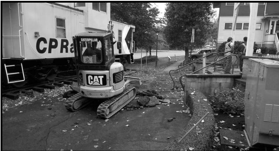
A small tracked excavator breaks up the asphalt in front of the Division's ex-CP caboose on October 7, to remove thick tree roots that had broken through the pavement. The area has since been repaved.
