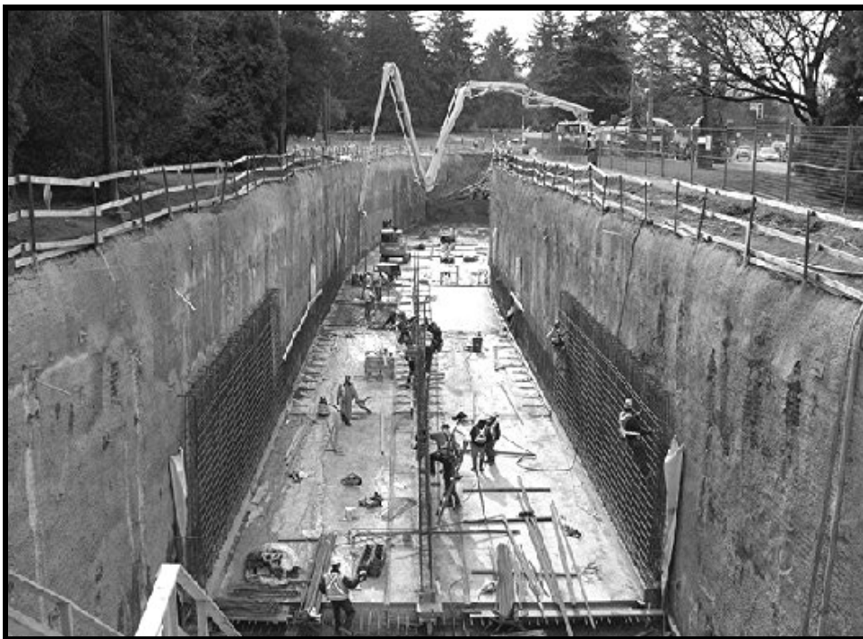
Looking south from 29th Avenue, this view shows cut-and-cover tunnel work on the alignment of the northbound lanes of Cambie Street. (Canada Line project photo)
