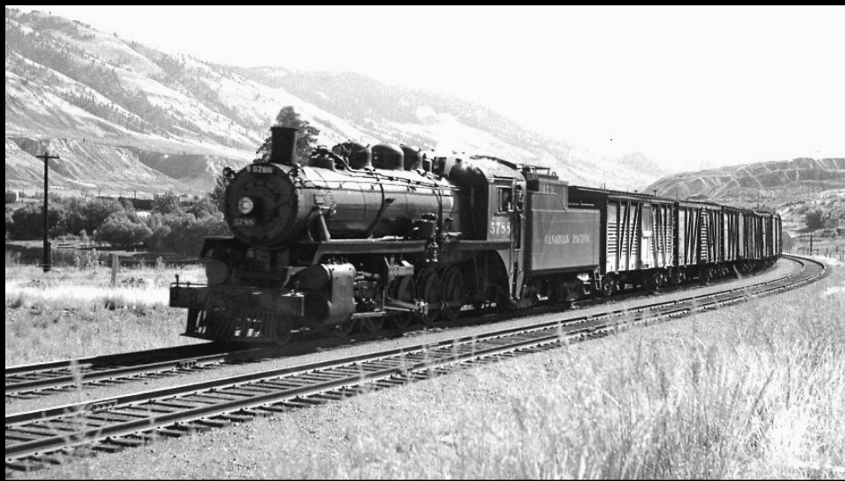
CP class R3d 2-10-0 locomotive 5788 approaches Kamloops yard with a westbound freight on August 1, 1945, with a stock car coupled to the tender.
