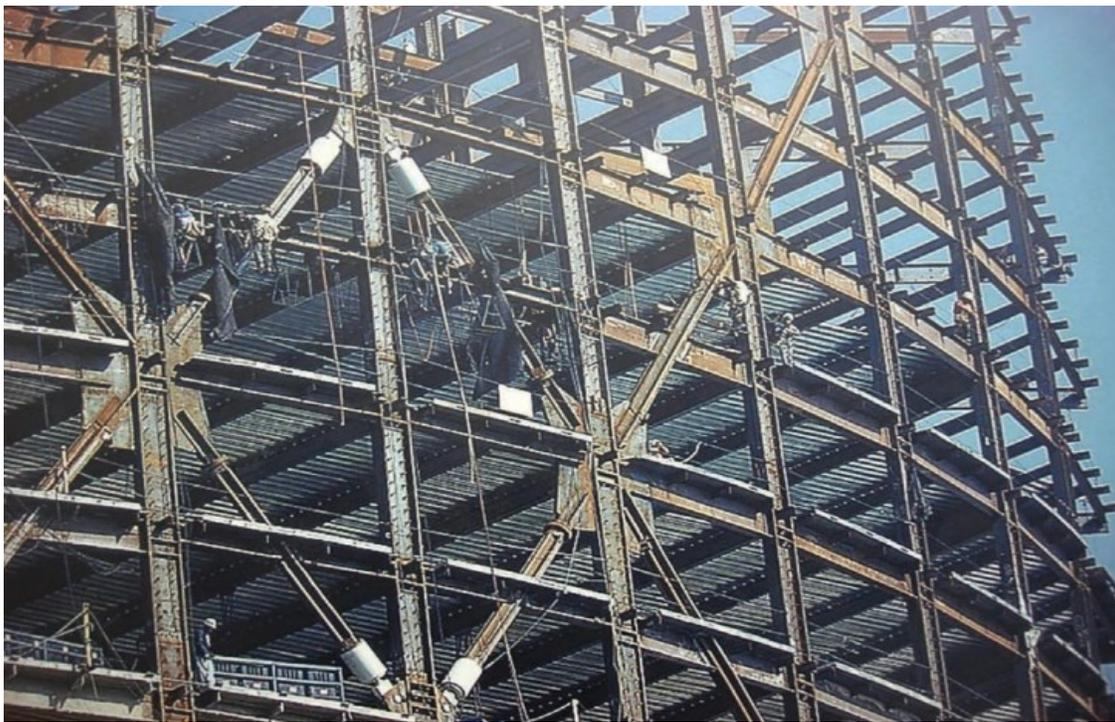
*Figure 52 Fluid Viscous Dampers in Diagonal Mega-Brace Configurations (Source: Taylor Devices).*
