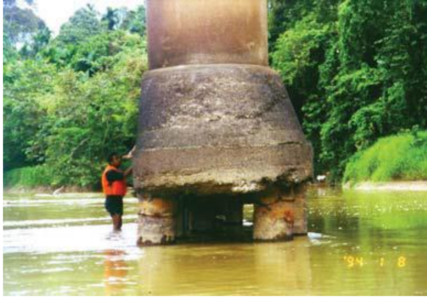
Figure 1–3: General scouring of river bed at Sg. Jeniang, Kedah
