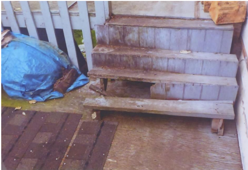
Image 4: rotten stairwell
