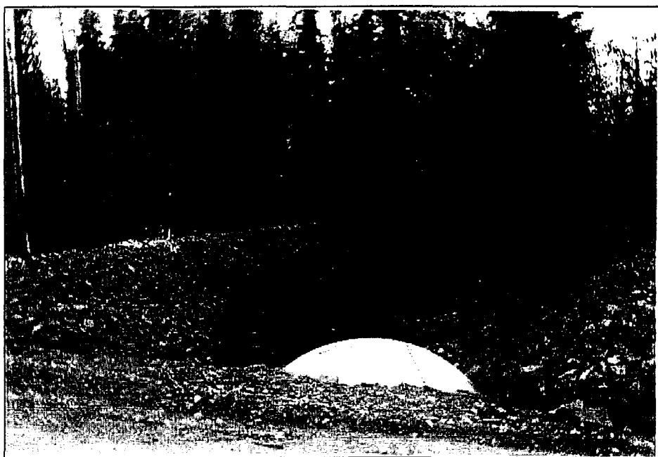
Photo 3.2: Upstream view of Cluculz Creek from the same location as Photo 3.1 showing the new pipe arch and the streambank revetment.
