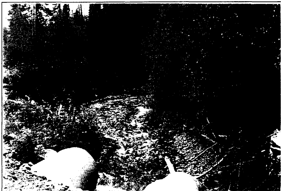
Photo 3.1 Upstream view of Cluculz Creek from the road showing the two culverts prior to their replacement with pipe arch and revetment of the streambank.
